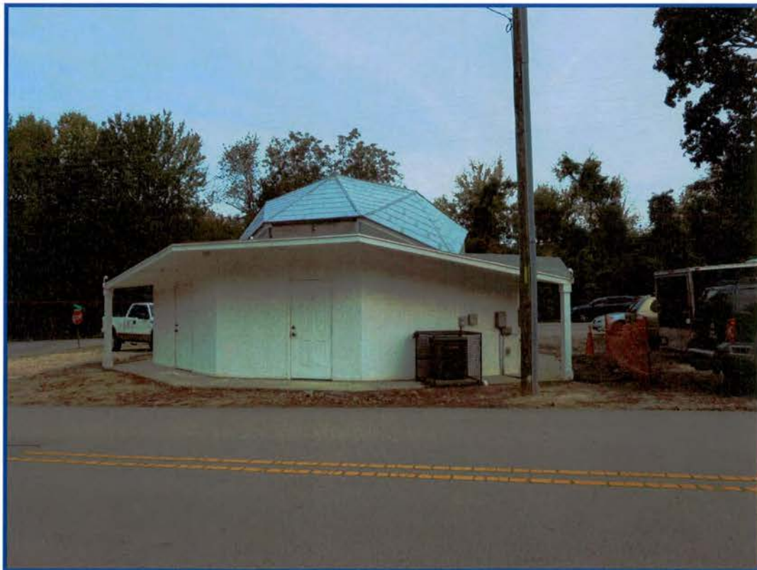
Looking N from Harwood Street
